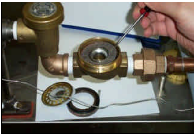
Removing the mesh strainer screen
